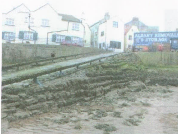
Photograph 3.14 Staithes 03-04-01. Cod & Lobster Slipway
