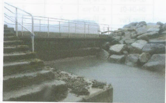
Photograph 3.21 Staithes Eastern Breakwater. Steps on eastern side.
