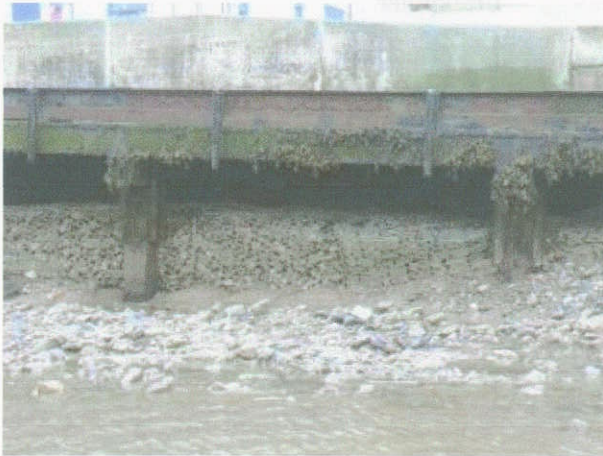
Photograph 3.10 Staithes RNLI Slipway. Gabion Baskets beneath slipway
