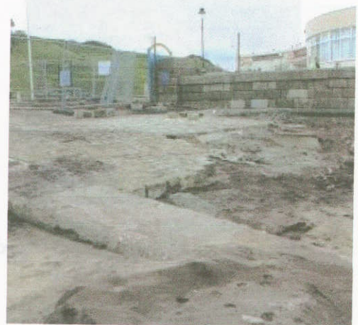
Photograph 3.71 SNB 43-20B-02. Works in progress
