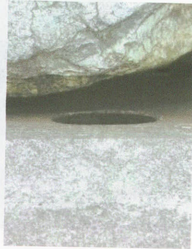
Photograph 3.54 Whitby West Cliff 18-11A-02 Drainage pipe
