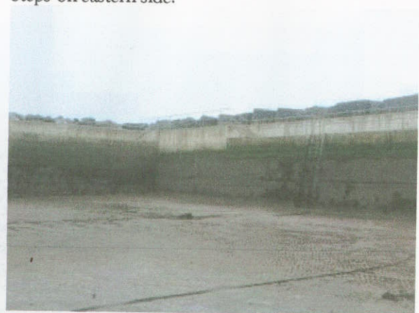
Photograph 3.23 Staithes Eastern Breakwater View on harbour side of concrete pier structure
