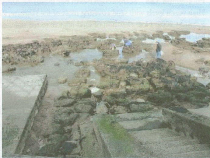
Photograph 3.73 SNB 43-20B-02. Works in progress
