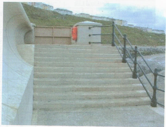
Photograph 3.75 SNB 46-20B-05. New defences have been constructed
