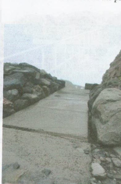
Photograph 3.2 Staithe Northern Breakwater. Slipway to Seaward side
