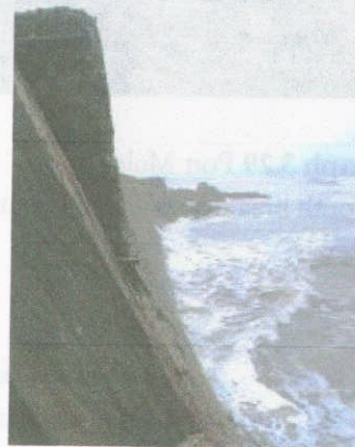
Photograph 3.27 Port Mulgrave. Seaward facing wall of south breakwater
