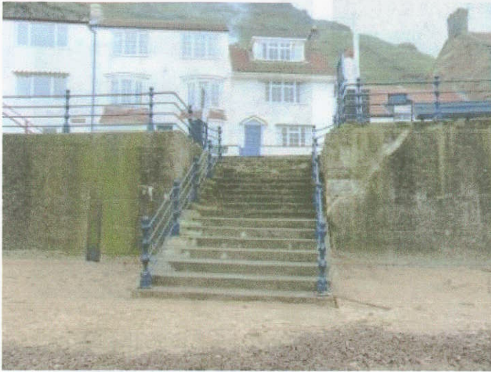
Photograph 3.16 Staithes 04-04-01. Steps and hand railing
