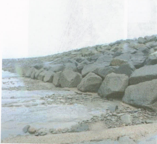
Photograph 3.1 Staithe Northern Breakwater. View at root of seaward revetment
