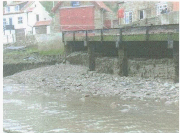
Photograph 3.11 Staithes RNLI Slipway. Gabion Baskets beneath slipway
