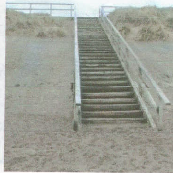
Photograph 3.46 Sandsend 16-09C-05 Staircase
