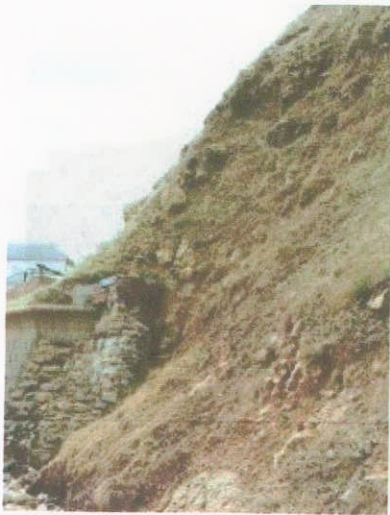
Photograph 3.85 Cayton Bay 58-24B-01. Steep coastal slope outflanking defence.
